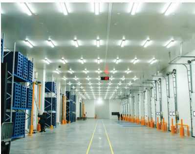
Cold Storage Warehouses
