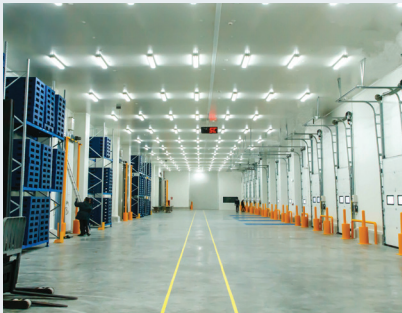
Cold Storage Warehouses
