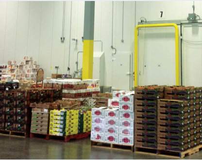
Medium to Large Warehouses
