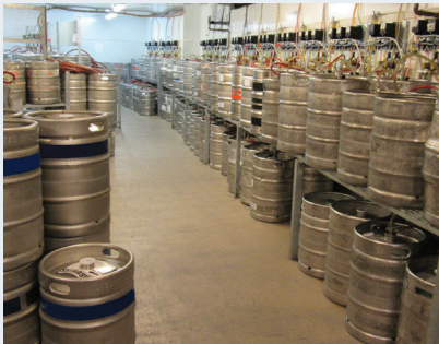
Walk-in Coolers and Freezers
