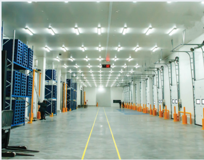
Cold Storage Warehouses
