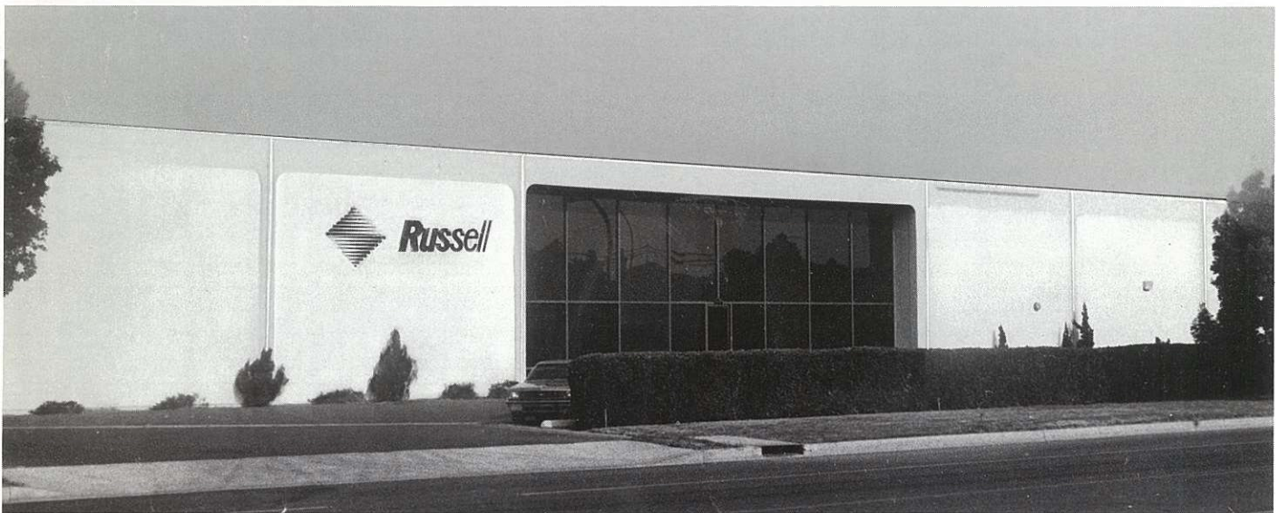
BREA, CALIFORNIA, EXECUTIVE OFFICES AND MANUFACTURING FACILITY
