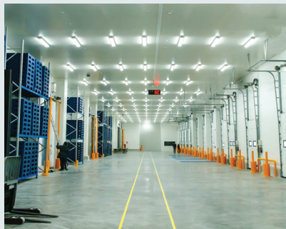
Cold Storage Warehouses
