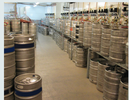
Walk-in Coolers and Freezers
